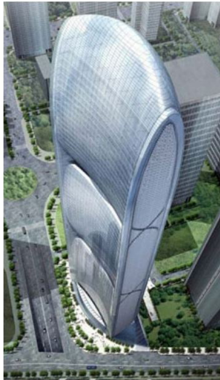
Figure 14: Zero-energy skyscraper «Pearl River Tower» [23] (spiral “wind vents” are visible on the right side of the house, solar panels are on the facade)
